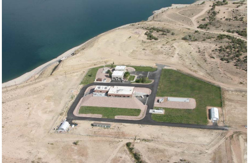
Duchesne Valley Water Treatment Plant
